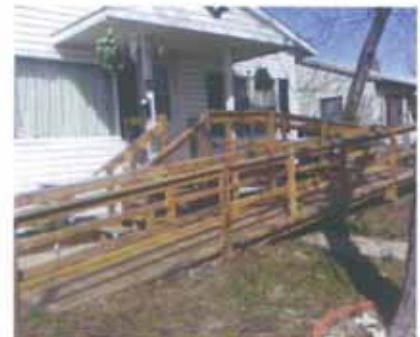
Keith's ramp paid for by CRP funds. His home is now accessible.
