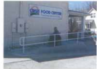
Cathy uses the new ramp at the Crisis Food Center.
